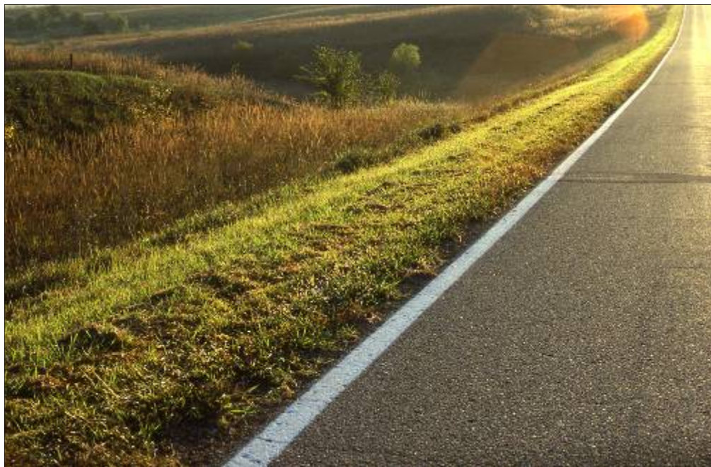
Mowing only a narrow road-edge strip can meet safety requirements and leave plenty of habitat. Photograph by Carl Kurtz.
